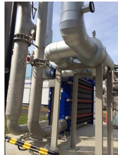
Reduction of Heating steam by heat exchanging between treated wastewater and industrial water
