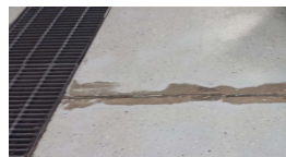
Above: Two examples of the common failures of coated floors. Chemicals have attack the drain area on the right, and movement of the concrete slab has made the coating crack and fail. These issues will do nothing but get worse over time.
