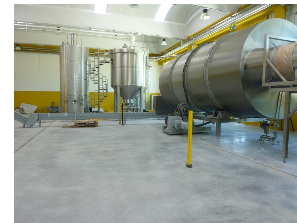
Picture 8: 10t Plant, Italy
